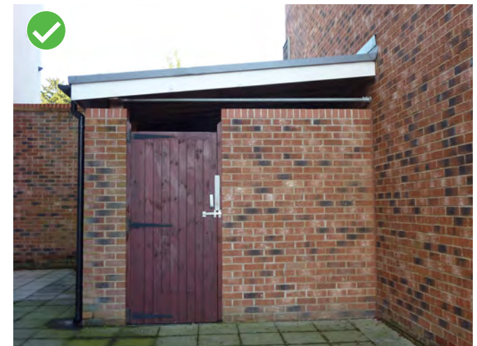
Below: Example of well considered storage design with robust, sturdy waterproof materials that compliment architecture.
